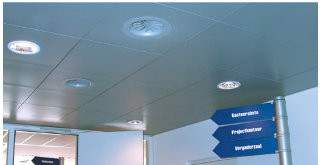
Triade Tower AMSTERDAM (Netherlands) Clip-in/hinge-down tiles in RAL 9006
