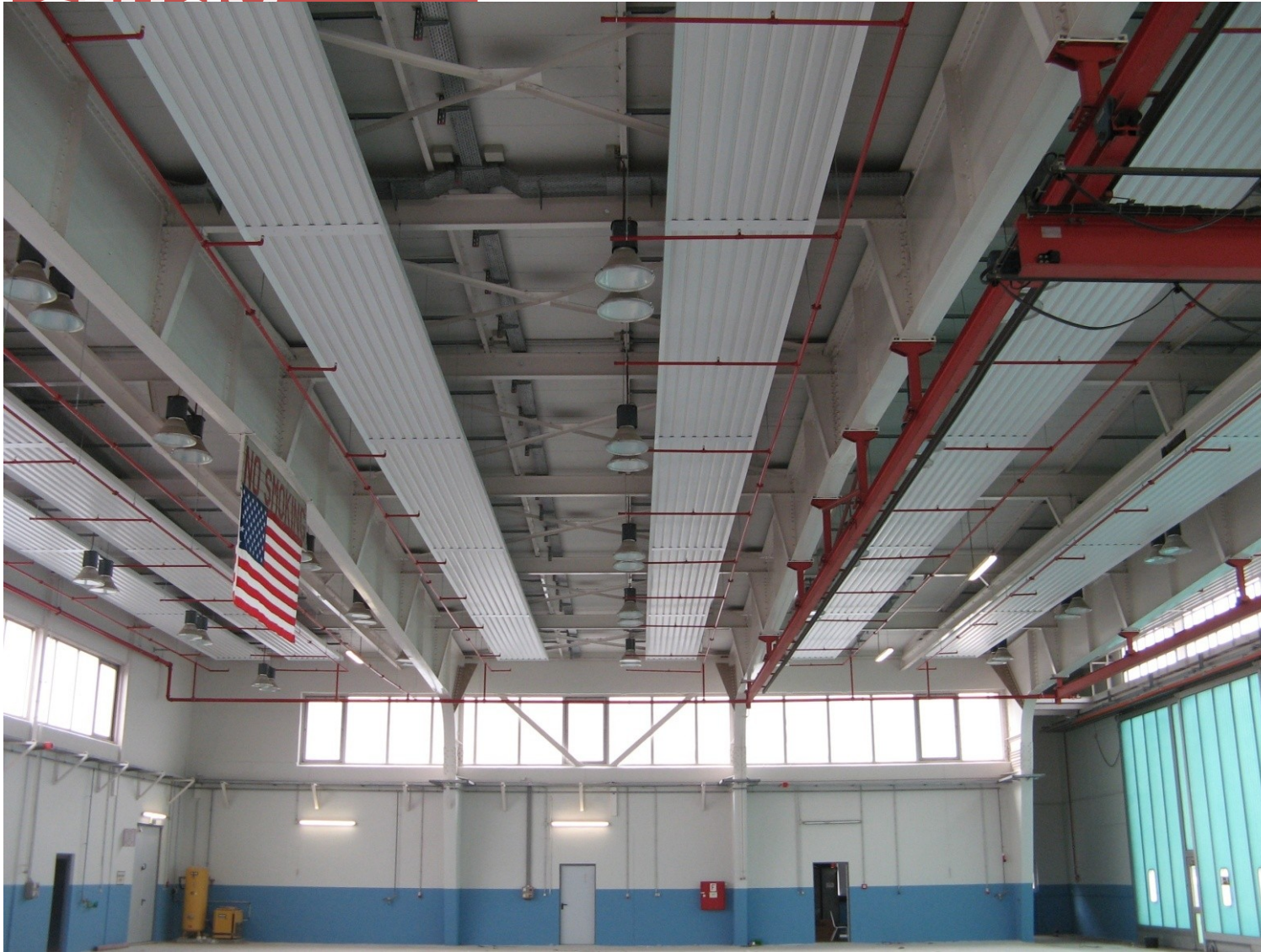
WAAF - Hangar 1035 FRENGER high efficiency radiant panel
