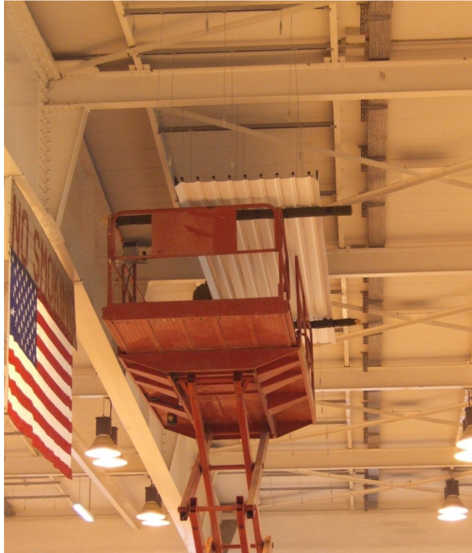
WAAF - Hangar 1035 FRENGER high efficiency radiant panel
