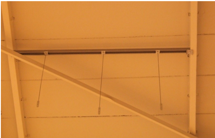
WAAF - Hangar 1035 FRENGER high efficiency radiant panel
